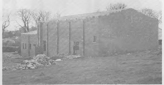
Community Centre nearing completion
